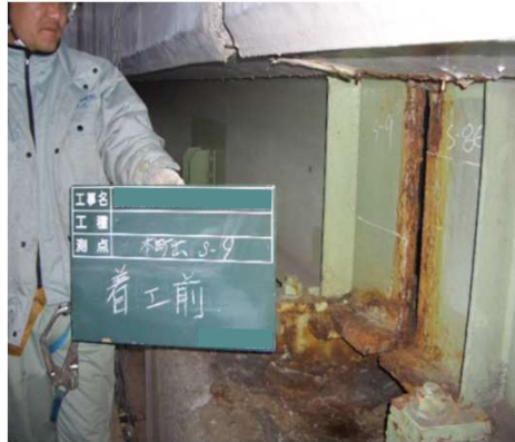
Corrosion of steel girder
