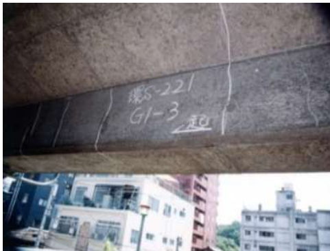
Crack of concrete girder
