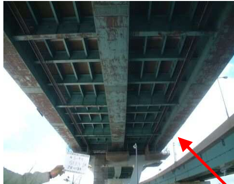
Deterioration of paint
