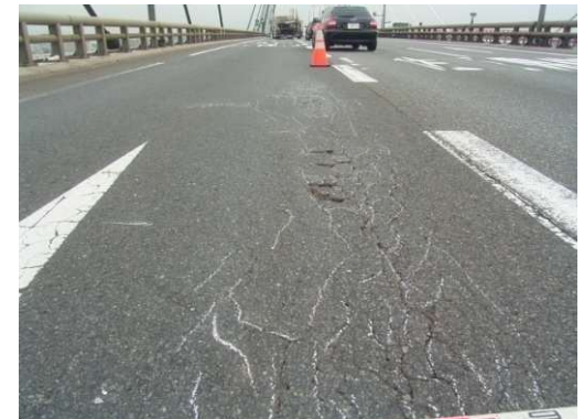
Deterioration of pavement
