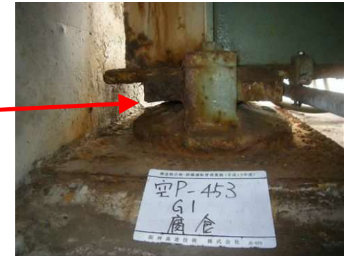
Rust of metal bearing
