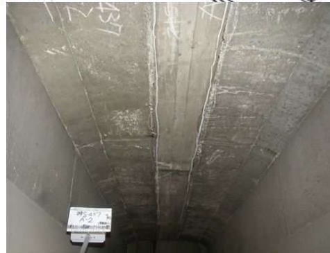
Crack of concrete girder
