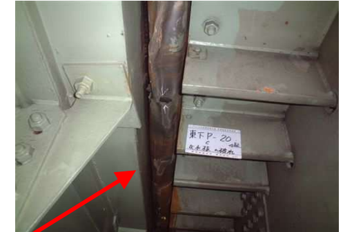
Damage of expansion joint
